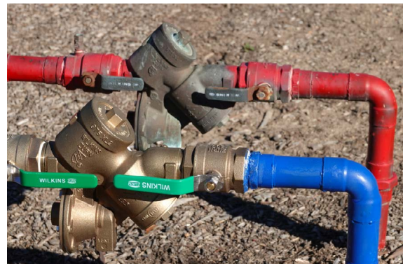
A backflow prevention device.
